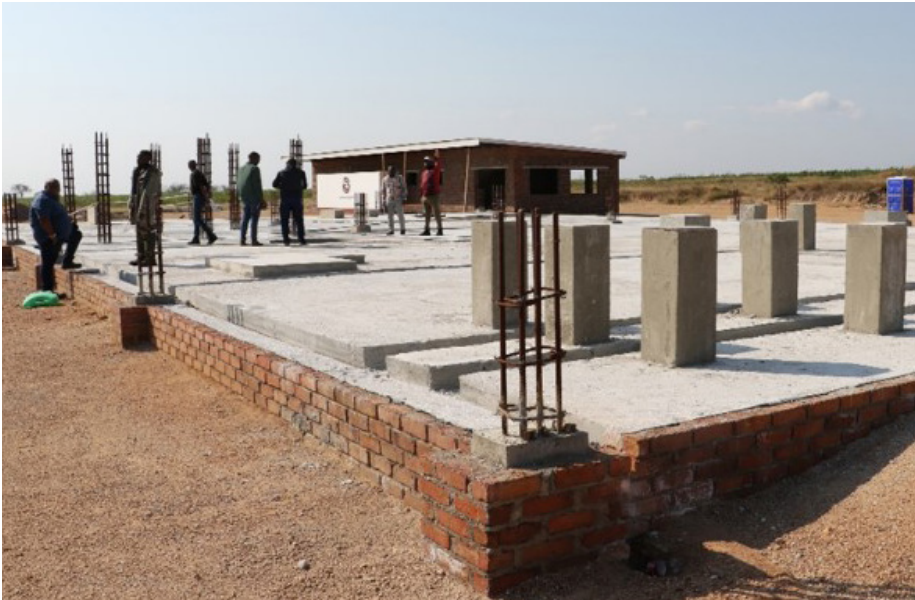
*Cassava processing plant under construction
